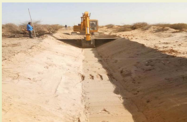
Drain Slope Cutting at Atndialakhar Site
